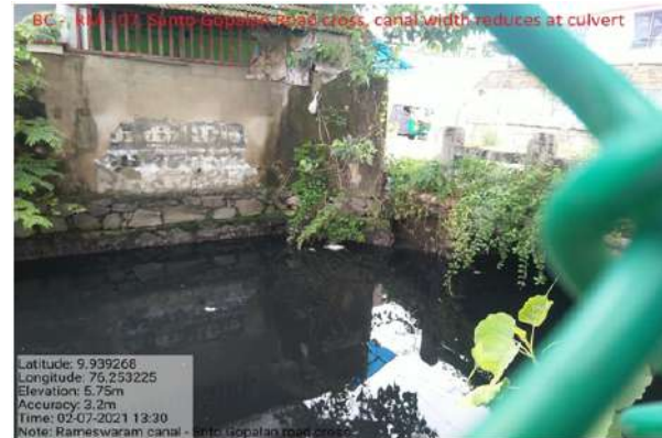
In ward No.25, at Ch. 1032m - Santo Gopalan Road cross canal width 7.50m, culvert span 5.50m
