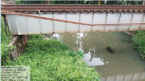
Chainage 36: Culvert have less vertical clearance, reconstruction of existing bridge is essential
