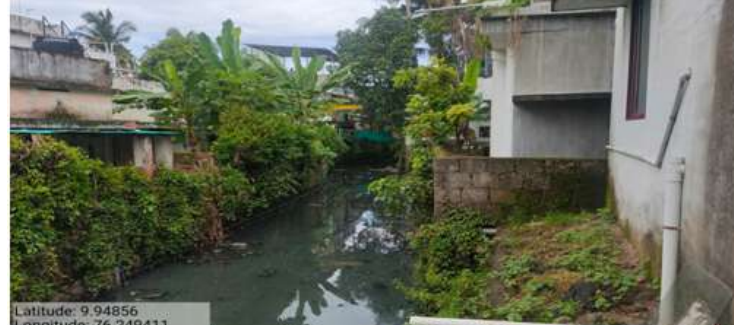
At. Ch.2972 - Heavy Silt deposit
