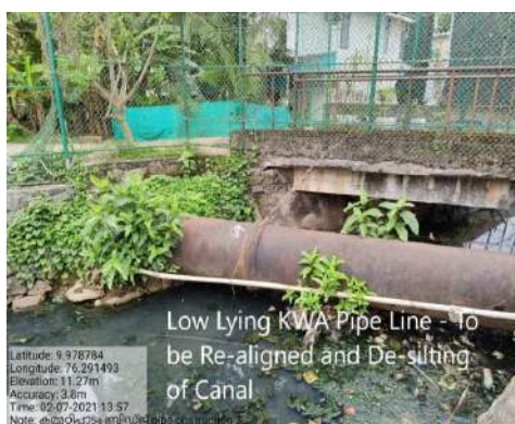
KWA Pipe Line to be Shifted
