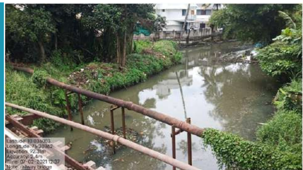
Chainage 1000: Covered with vegetation on both banks, Disposal of waste and silt deposition
