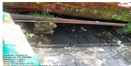
In Ward No.8, at Ch. 2873m Pandikudy Bridge , Beam soffit touching the water and KWA pipe line with additional two pillars
