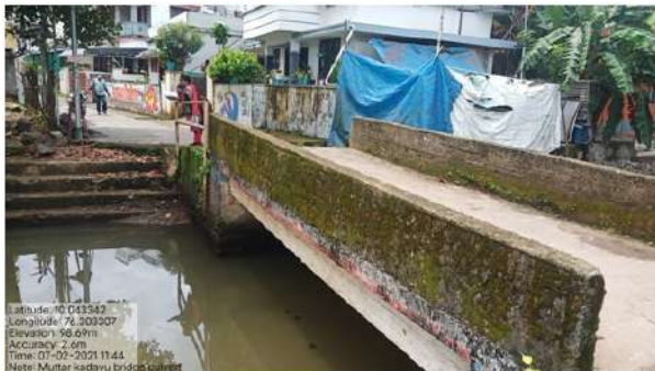
Chainage 36: Culvert have less vertical clearance, reconstruction of existing bridge is essential
