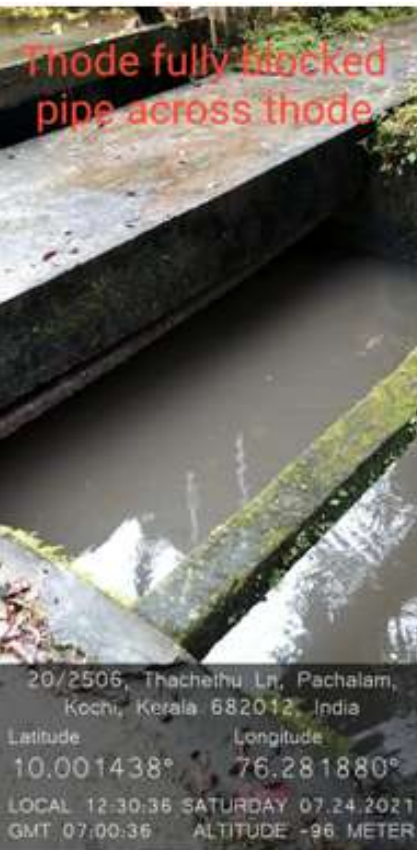
8. At Ch 840 m - culvert fully blocked, pipe across thode.
