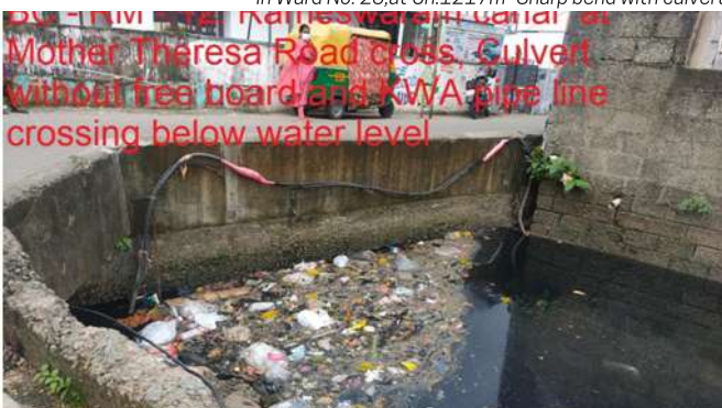
In Ward No.8, at Ch. 1758m Mother Theresa Road cross - culvert without free board and KWA pipe line crossing below water level
