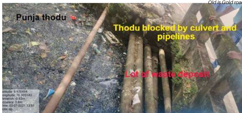
Thodu blocked by culvert and pipelines
