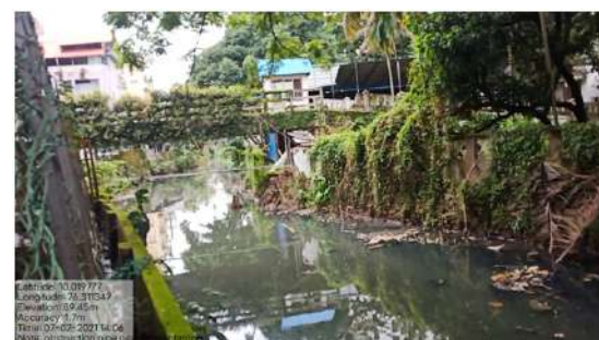
1" water line pipe laid across the thodu is found to obstruct the flow, deposition of silt is noticed.
