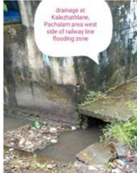
16. West side of railway line at Kalezhath Ln. Railway culvert blocked Kalazhath Ln. flooding area near Pachalam market
