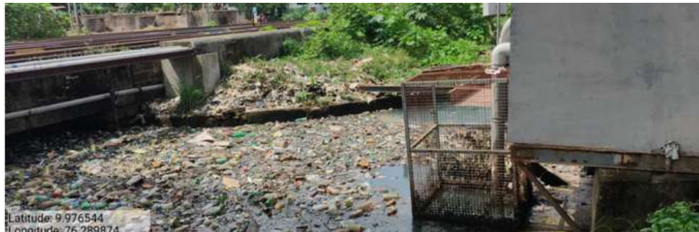
OBSTRUCTED RAIL CULVERT NEAR STARTING POINT OF MULLASSERY CANAL
