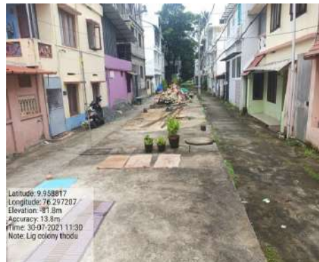
LIG Colony Thodu – Covered with Concrete Slabs – To be opened
