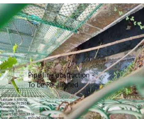
KWA Pipe Line to be Shifted and CD Works to be Re-constructed
