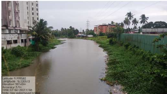
Chainage 7200: Vegetation on both banks, accumulated with floating wastes and is covered with hyacinth.
