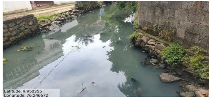
At. Ch.3599 - Heavy Silt deposit
