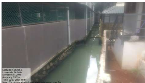
Reach behind NOEL Apartment- Insufficient width and passing between compound walls
