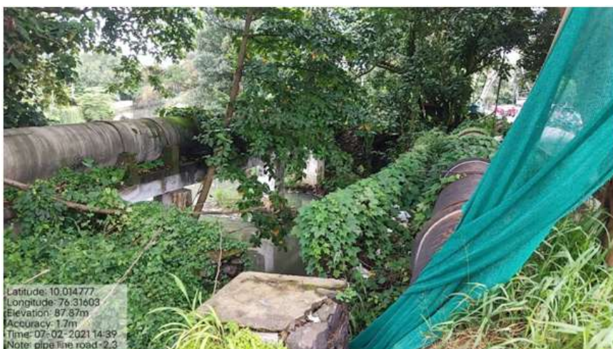
Chainage 3230 : Covered with vegetation on both banks, accumulation of silt
