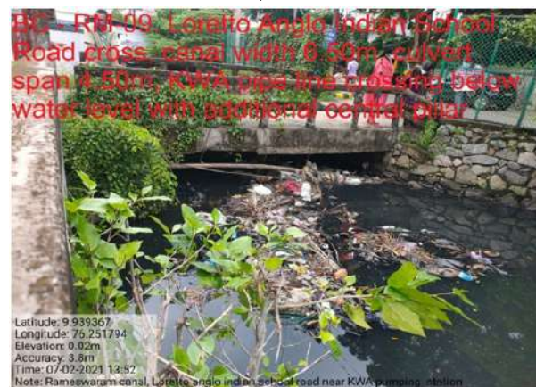
In Ward No. 25, at Ch. 1190m - Loretto Anglo Indian School Road cross, Canal width 6.50m and culvert span 4.50m
