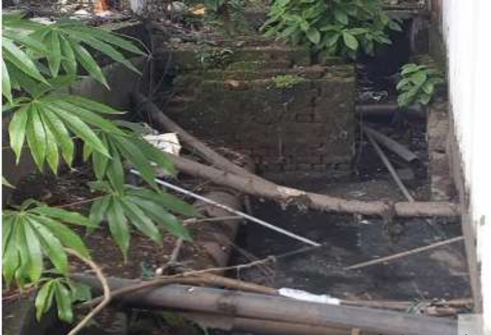
Choked leading drain outside the entrance of substation that supposed to lead water from Changadompokku to Karanakodam
