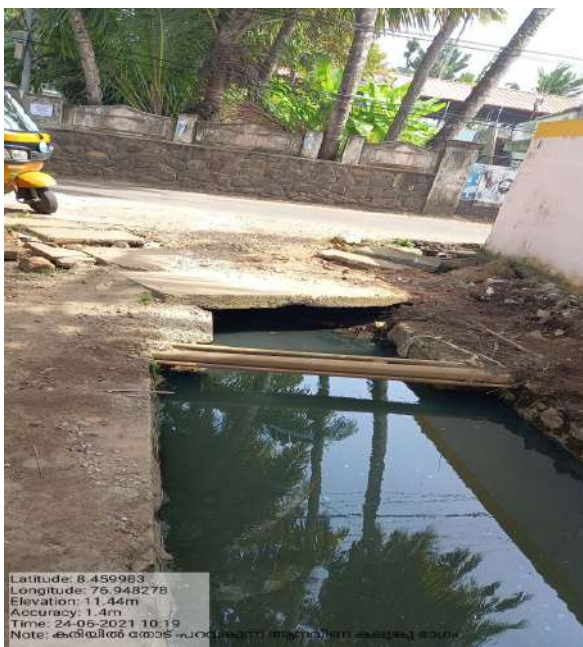
Kariyil thodu Paravankunnu @ Anaveena Kalungu (solution - Desiltation & Widening & rising of culvert)
