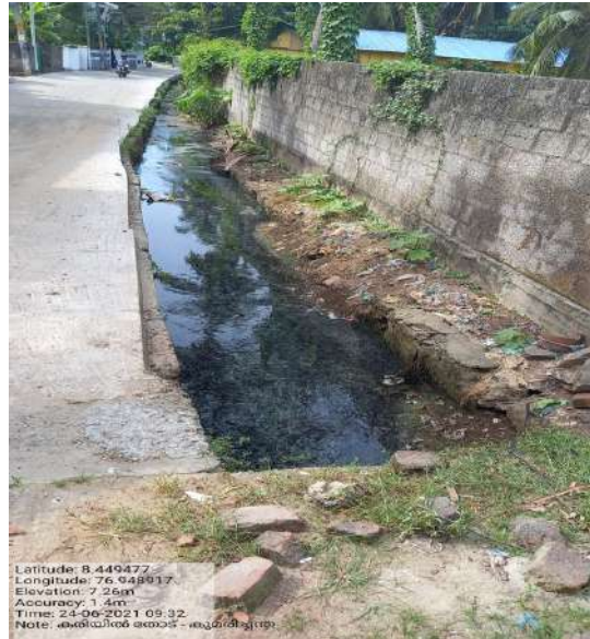
Kariyil thodu@ Kumarichantha south side (Encroachments & high siltation)
