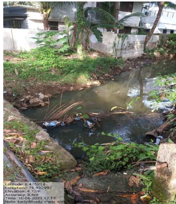
Kariyil thodu @ meeting point with Theckanakkara canal (With waste and silt ,-flow obstructed)
