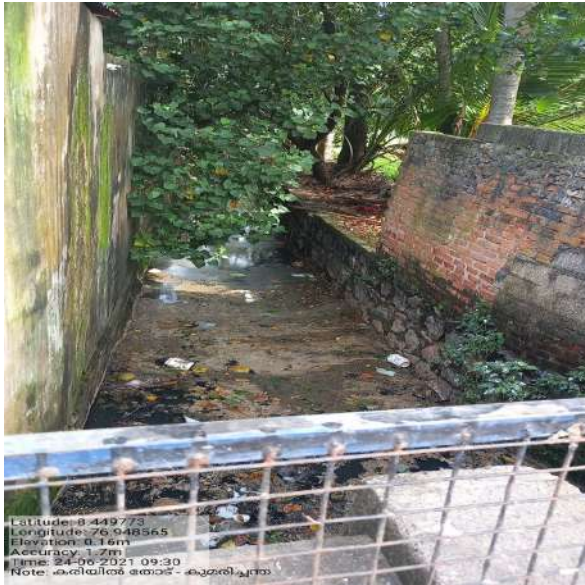
Kariyil thodu@ Kumarichantha (Siltation & Waste dumping is main problem)
