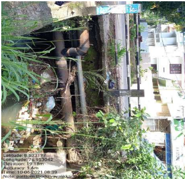
Pattom Thodu @ Vayalikkada Bridge (Blokage due to low level crossing of service lines)
