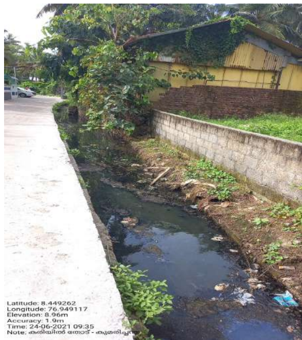
Kariyil thodu @South of Kumarichantha ( Siltation & Vegetation to be removed )
