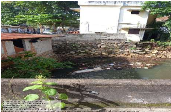
Pattomthodu @U/S of Pattomthanupillai bridge portion (High siltation Waste deposit )
