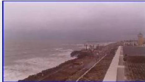
Sea wall protection
