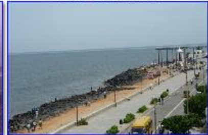
Strengthened sea wall
