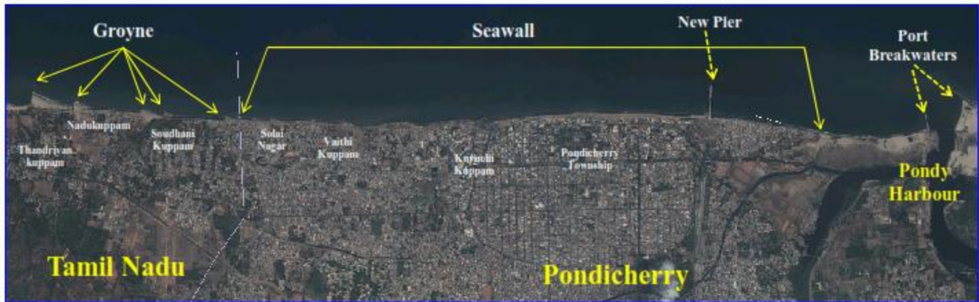
Coastal Structures along Pondicherry
