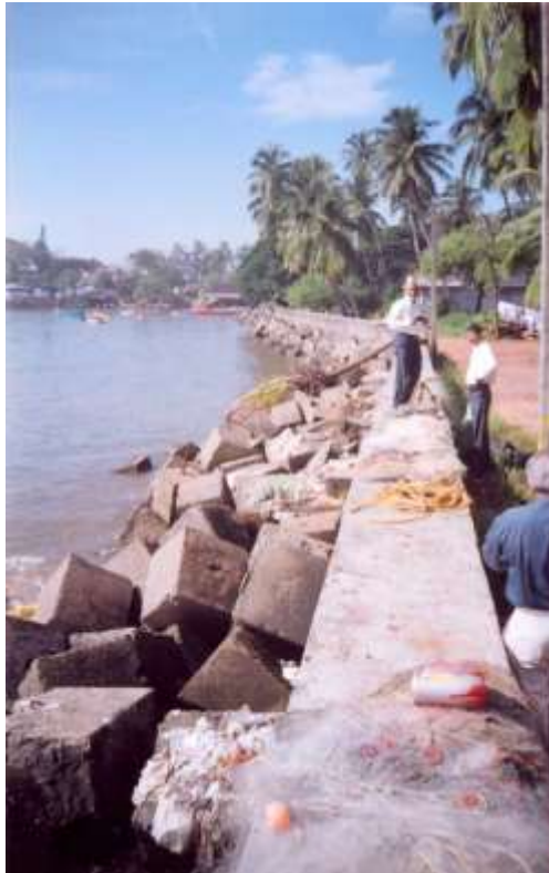
Figure 1.2.3. Revetment along Dona Paula, Goa Coast
