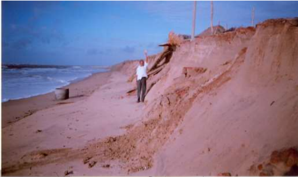
(a) Sand dune erosion at Paradip, Orissa.
