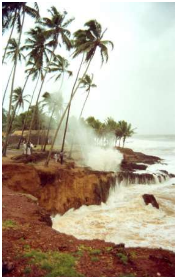
(b) Cliff erosion at Anjuna, Goa.
