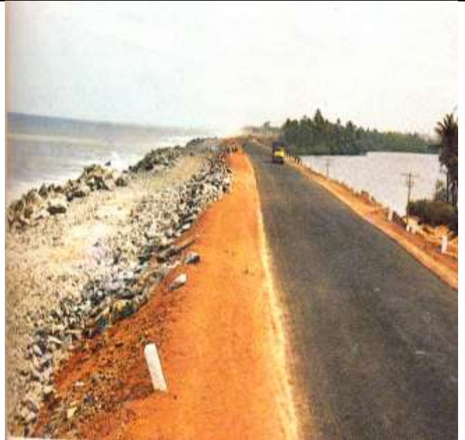
(b) Seawall at Maravanthe, Karnataka
