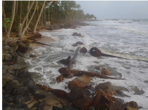
Figure 7. Erosion at Chenneveli (north of Chethi harbour)
