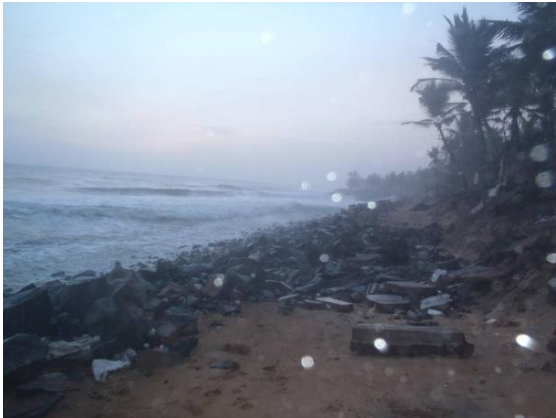
Figure 2. Damaged Seawall at Bhimapally
