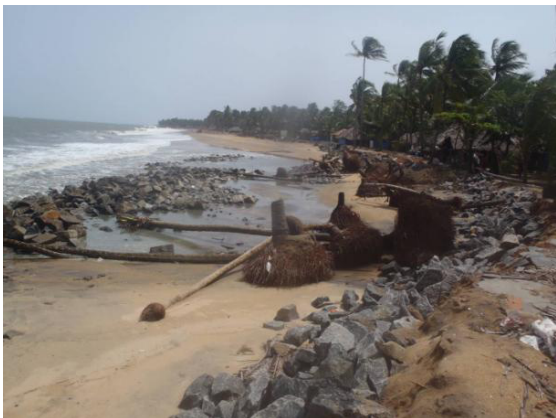
Figure 8. Erosion at Puduponnani
