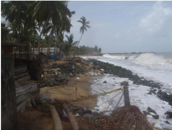
Figure 6. Erosion at Thanoor (north of breakwater)
