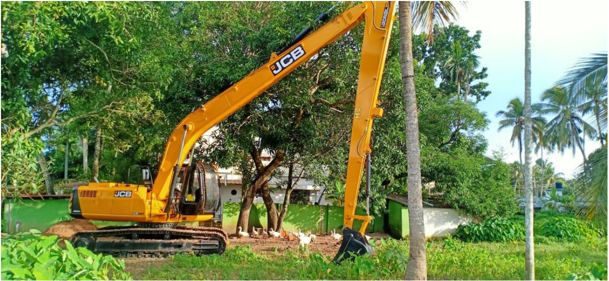
Long Reach Excavator
